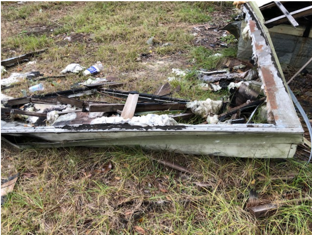
This photo depicts remnant silver coating from the damaged roof.
