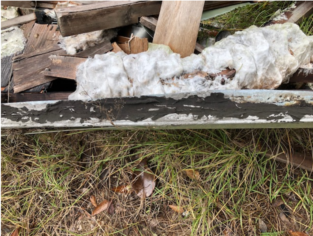
This photo depicts the silver coating and tar sampled from the remnant roof.
