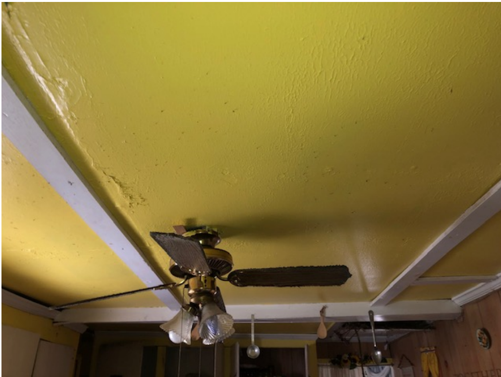
This photo depicts the ceiling in the kitchen.
