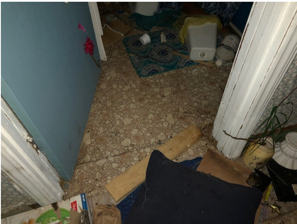
This photo depicts the sheet flooring sampled from the bathroom.
