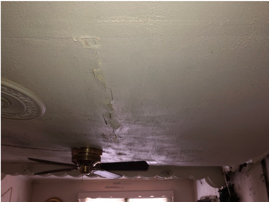
This photo depicts the ceiling texture in the living room.
