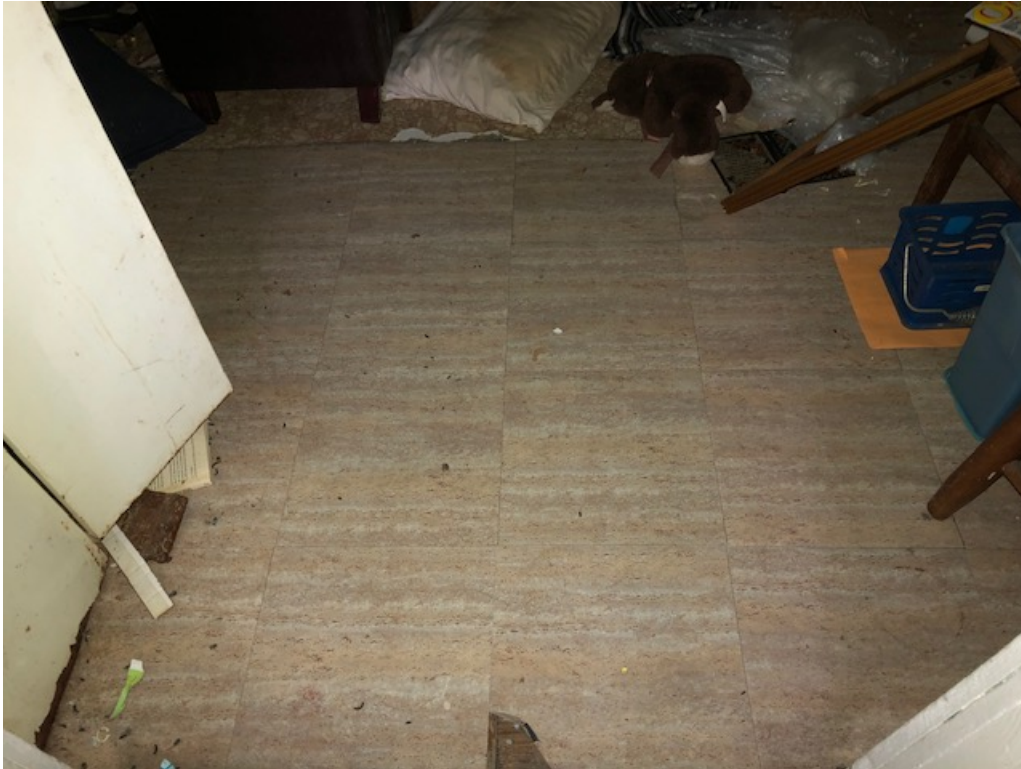
This photo depicts the floor tile in bedroom 1.
