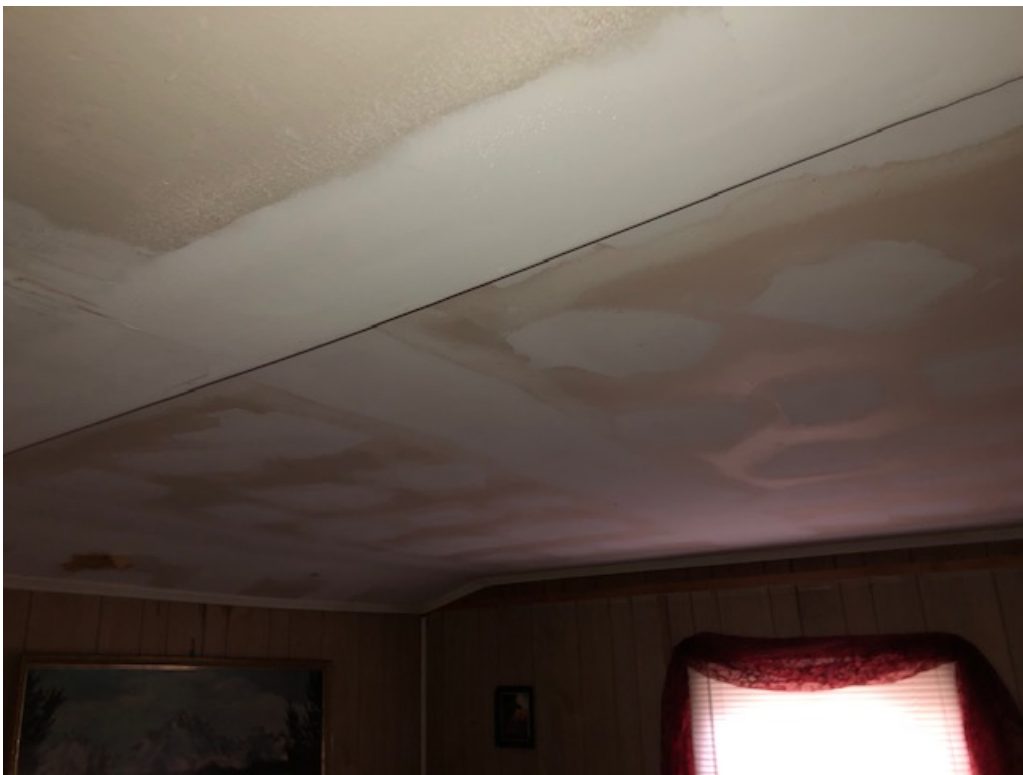
This photo depicts a view of the ceiling in the bedroom.
