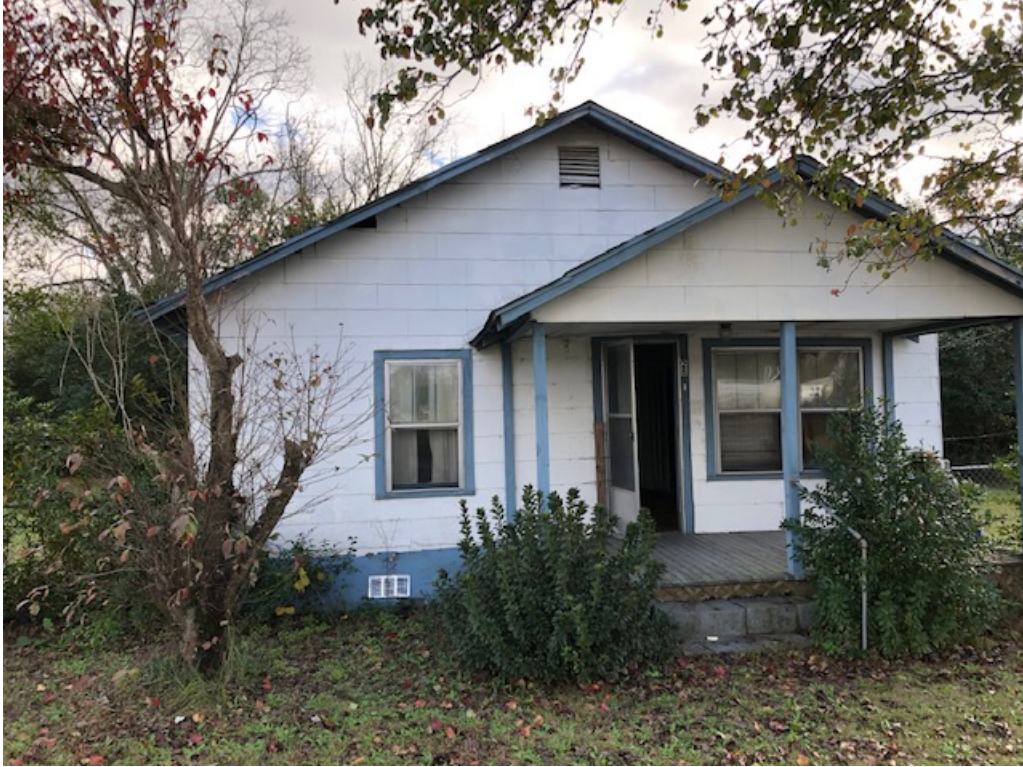
This photo depicts the front of the residence.
