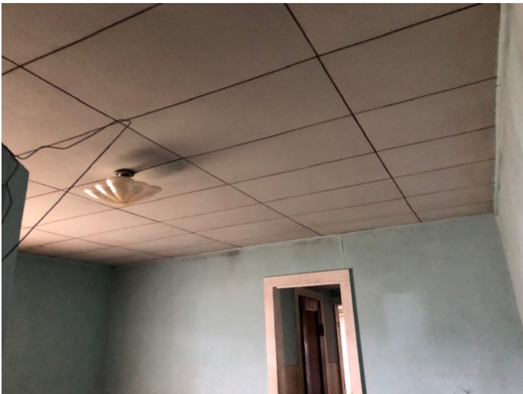
This photo depicts the ceiling tiles sampled from bedroom 2.
