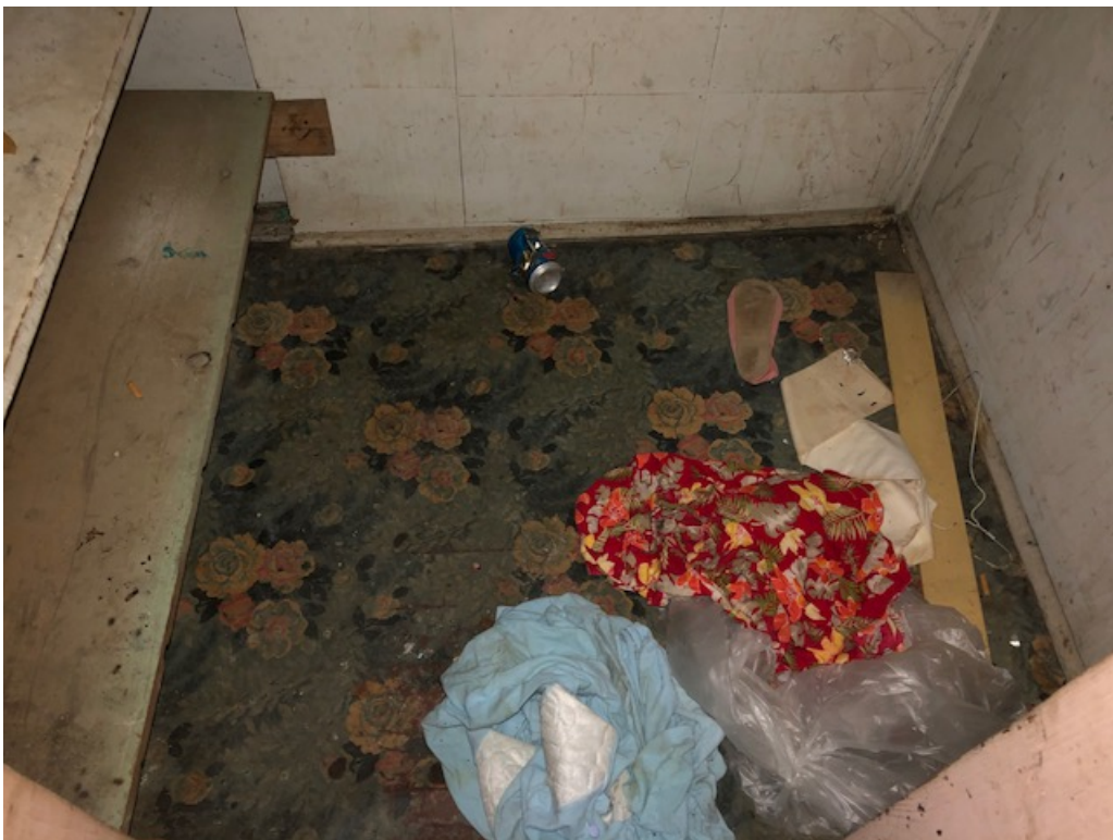
This photo depicts the sheet flooring sampled from the closet.
