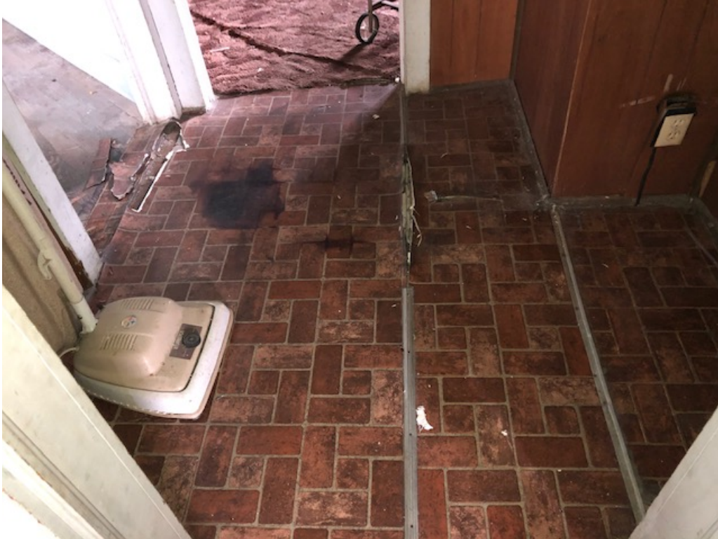
This photo depicts the sheet flooring sampled from the hallway.
