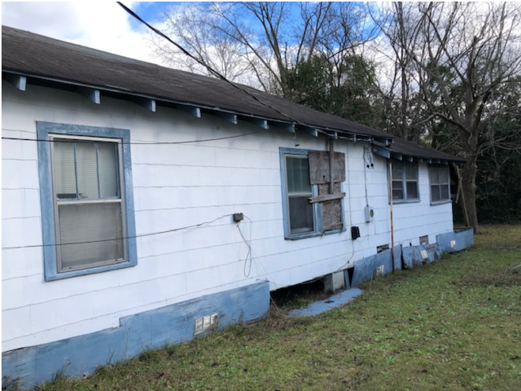
This photo depicts the side of the residence where transite was sampled.
