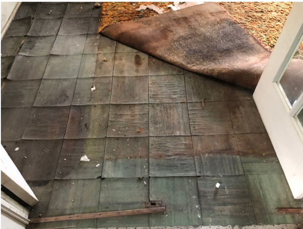
This photo depicts the green floor tiles sampled from the living room.
