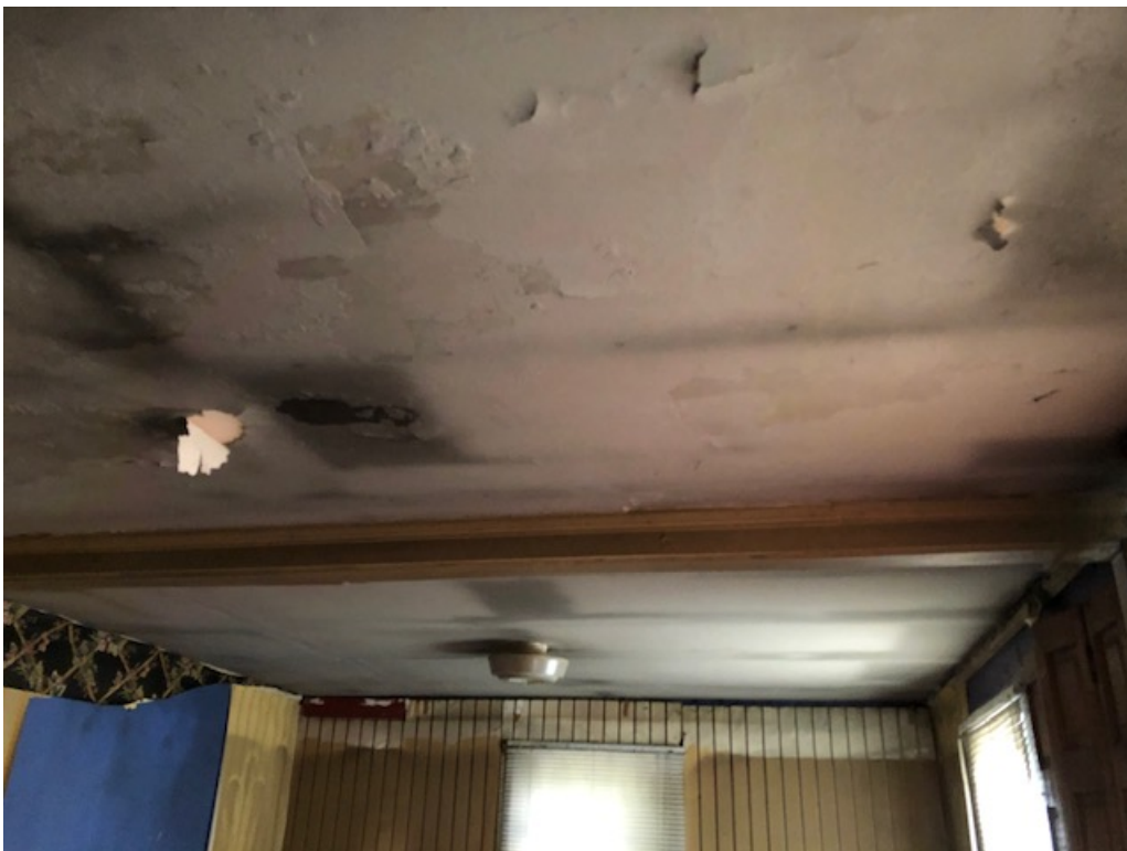
This photo depicts the ceiling in the living room where drywall joint compound was sampled.
